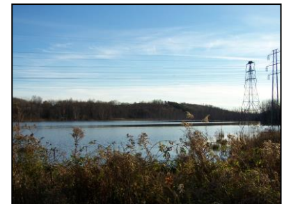
Powers Road Wetland, facing south towards the Town of Throop. Osprey nest is visible on top of left electrical tower.
